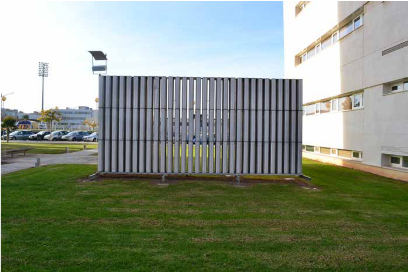
Figure 6: Sonic crystal noise barrier created by the Wave Phenomena Group, Polytechnic University of Valencia, Spain. Source: Reprinted from García-Chocano, V., Cabrera, S. & Sánchez-Dehesa, J. (2012) Broadband sound absorption by lattices of microperforated cylindrical shells. Applied Physics Letters . 101 (18), pp. 184101, with the permission of AIP Publishing.
